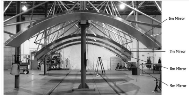
Fig. 6: Mirror panels of different aperture width installed on a space frame at the SkyFuel Development Test Center.
