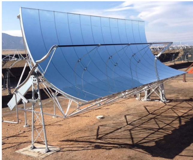
Fig. 1: Full scale single module (7.6m aperture x 18.5m length) SkyTrough® DSP.
