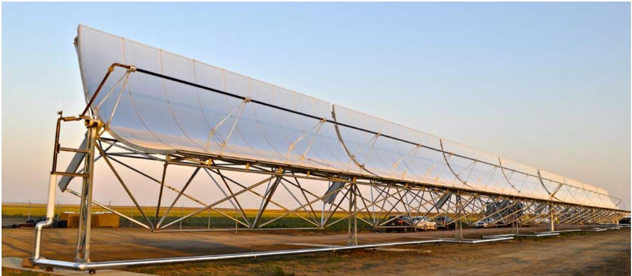
*SkyFuel's high performance, low cost SkyTrough® parabolic trough solar collector, supplying heat to WaterFX desalination system .*
