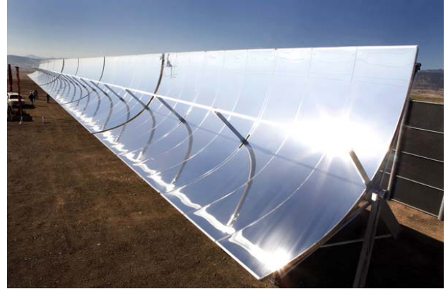
Figure 7 - SCA Installed and Tracking the Sun
