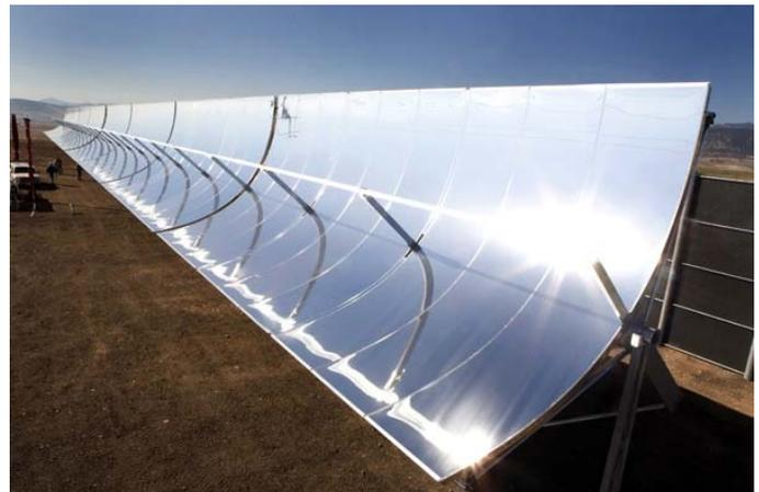
**Figure 1 – SkyTrough™ SCA, Tracking the Sun**
