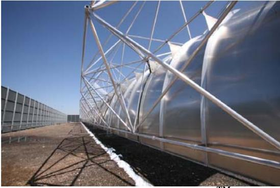
**Figure 2 – back side view of the SkyTrough™ space frame**
